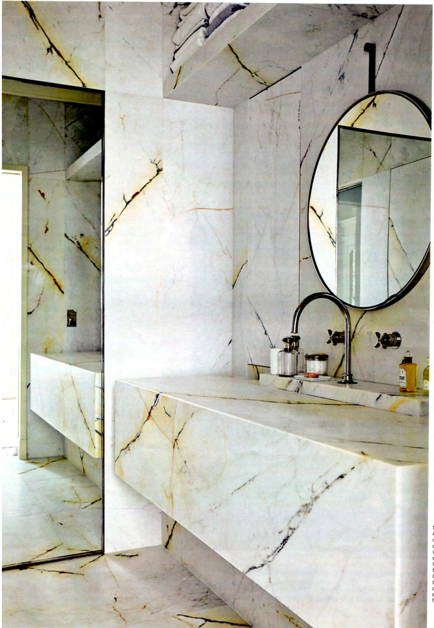
STONE AGE A massive block of marble has only the slightest indent for the sink, with Waterworks fixtures. Concealed between the slab and the wall is an open space for storage.
